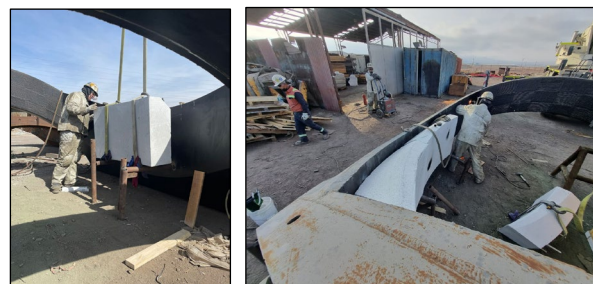
Installation of precast shapes.
