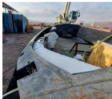
Installed METAL-ROK® Precast
