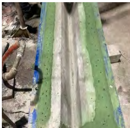
Installed precast insert
