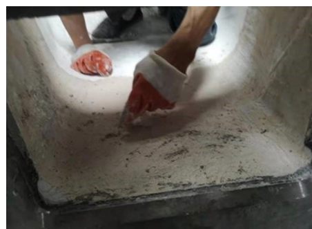
Spout repair using QUICK-FIRE® ONE 86
