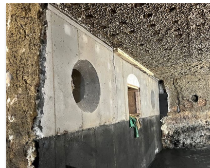
Burner wall after form removal
