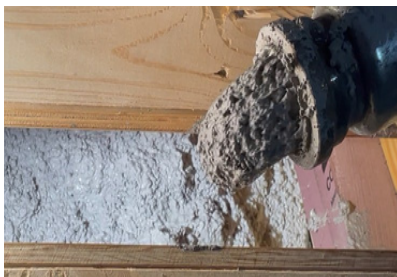
Pumping MATRIFLO 80 ACX PUMP into Forms
