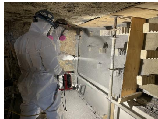
Gunning REDIGUN 85 P in Upper Wall
