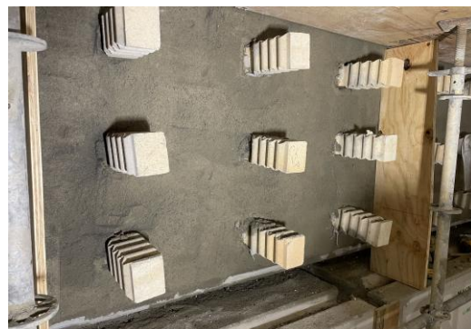
Ceramic Anchors placed in Upper Wall
