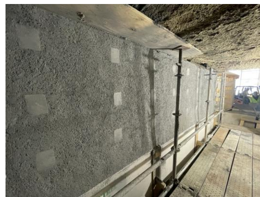
REDIGUN 85 P Installed as Working Lining
