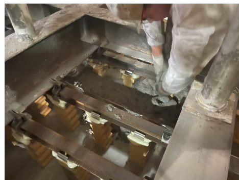
NANO-TEK® 70 pumped on the roof
