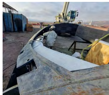
Installed METAL-ROK® Precast
