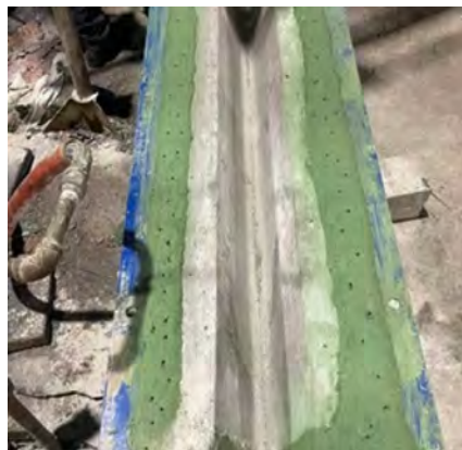
Installed precast insert
