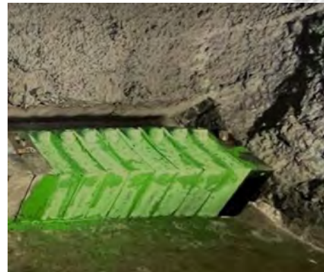
Tuyere System installed with Peirce-Smith Converter
