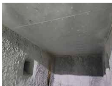
Inside furnace after forms were pulled
