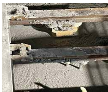
Material being pumped
