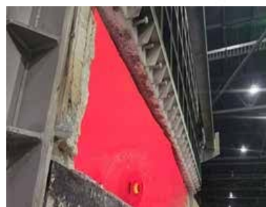
Roof after heat up
