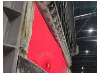
Roof after heat up
