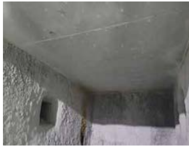
Inside furnace after forms were pulled
