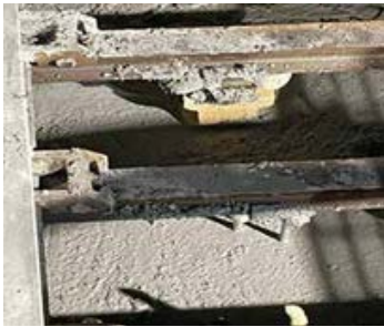
Material being pumped
