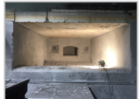
QUICK-FIRE® 88 installed
