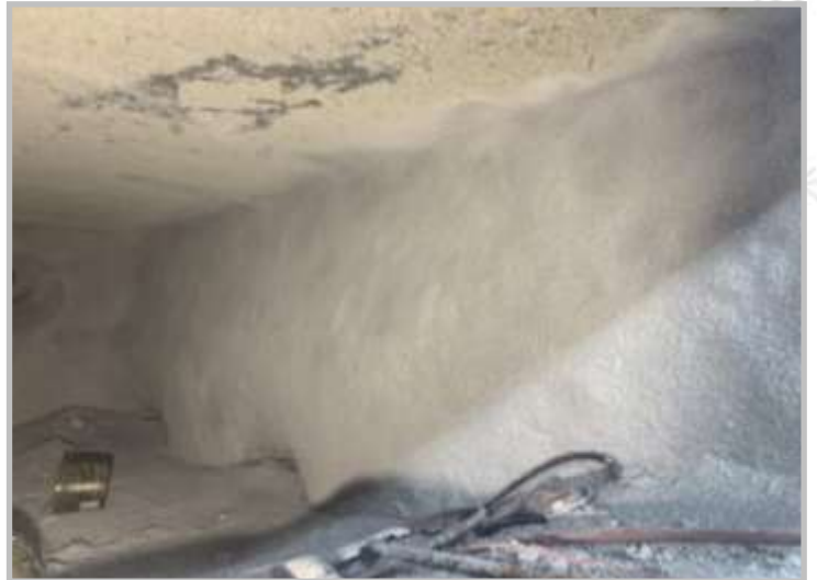
AFTER: QUICK-FIRE® ONE 84 G installation completed
