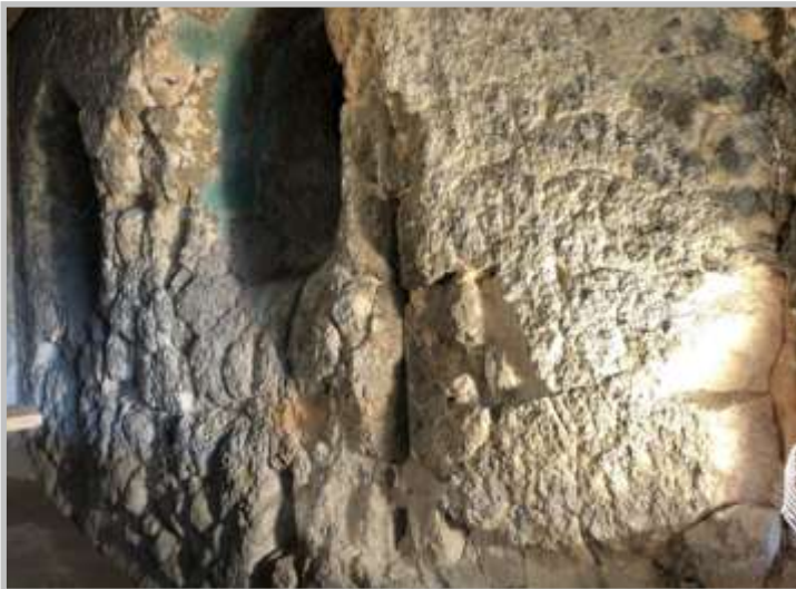
BEFORE: Furnace with material needing repair
