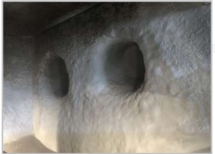
AFTER: QUICK-FIRE® 85 G installation completed
