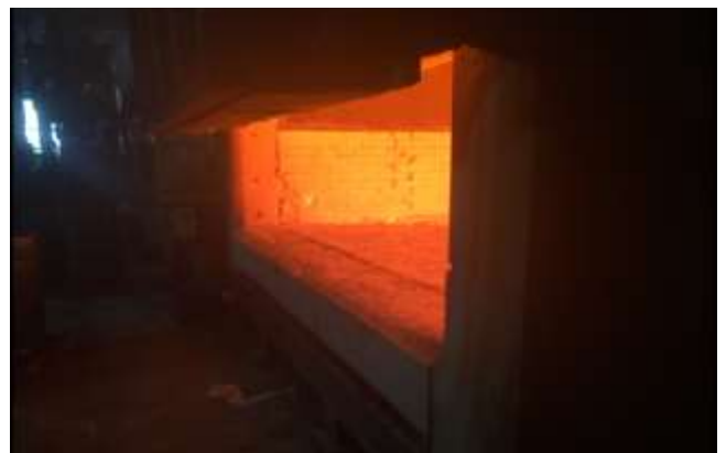
ARMORMAX® sill after 52 months in service
