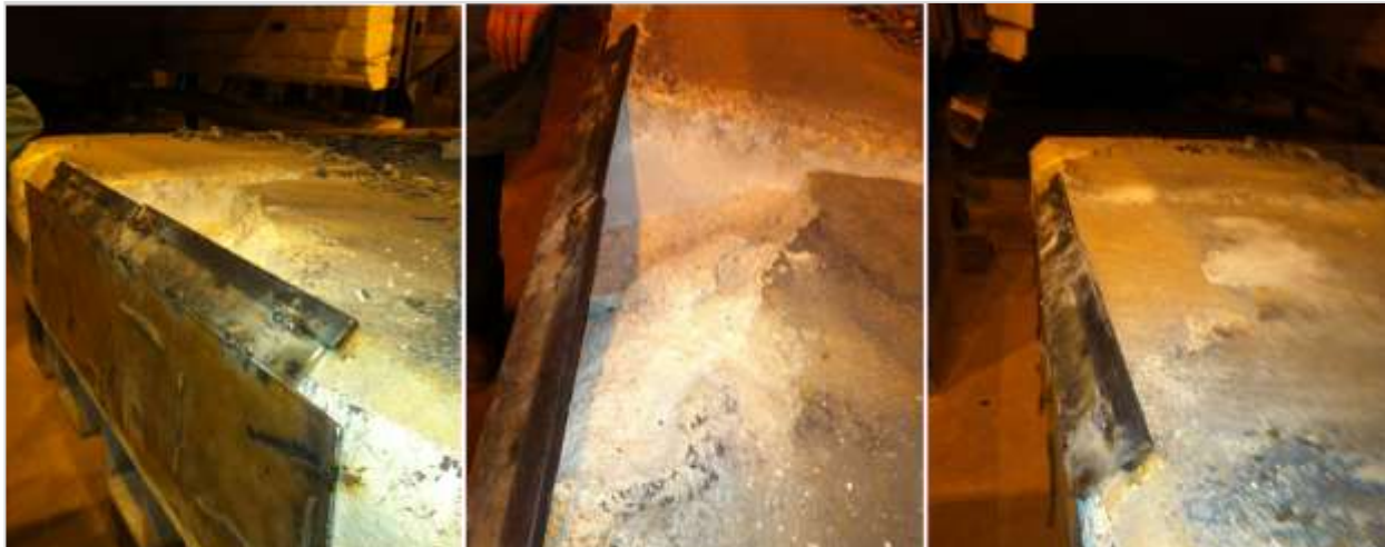
QUICK-FIRE® 65 perimeter repair
