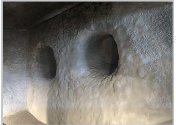
AFTER: QUICK-FIRE® 85 G installation completed
