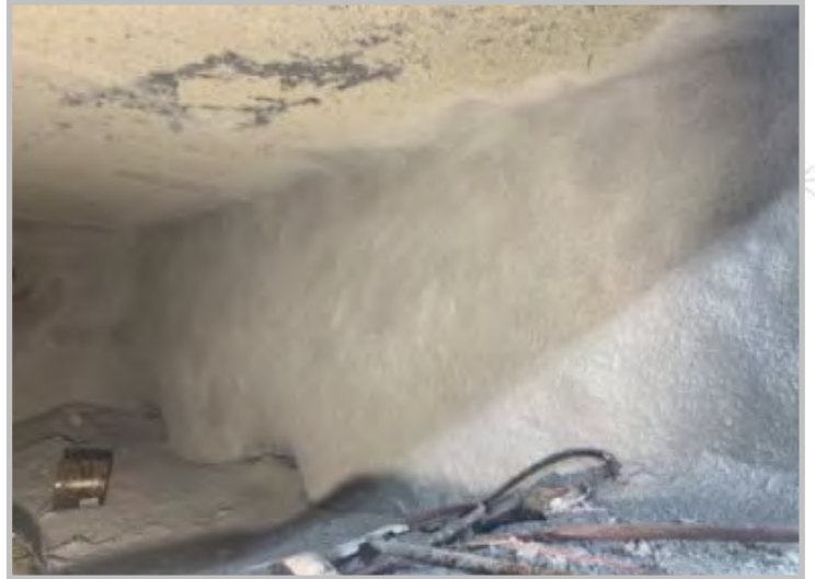
AFTER: QUICK-FIRE® ONE 84 G installation completed
