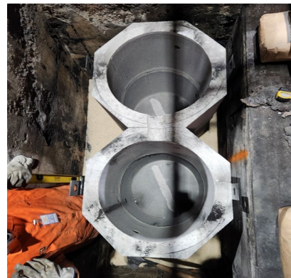
Modules set in place
