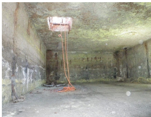
Sulfur Pit (Before)
