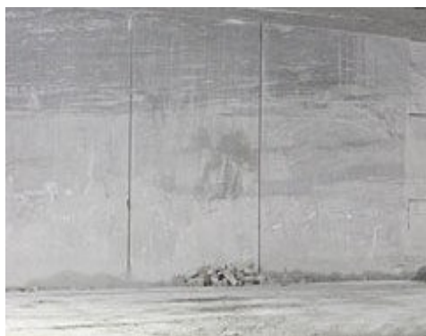
Sulfur Pit (After)
