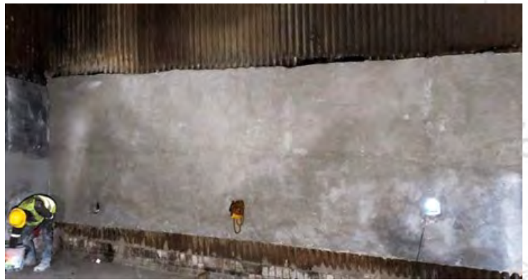
AFTER: QUICK-FIRE® PATCH M
