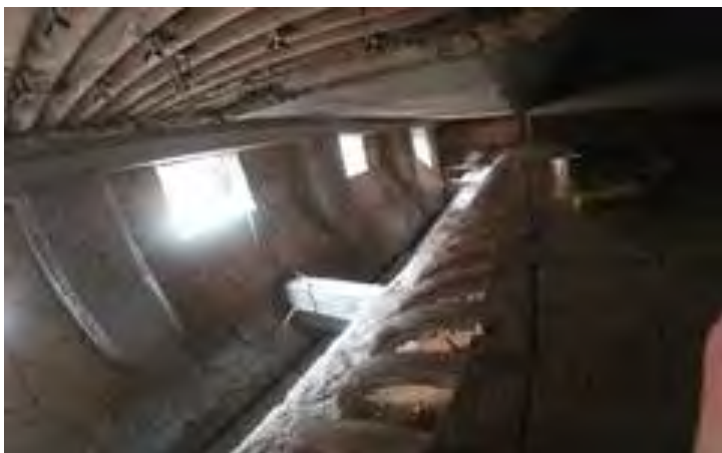
BEFORE: Installation of QUICK-FIRE® PATCH M
