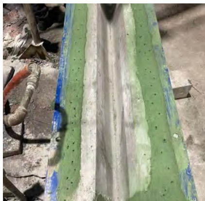
Installed precast insert
