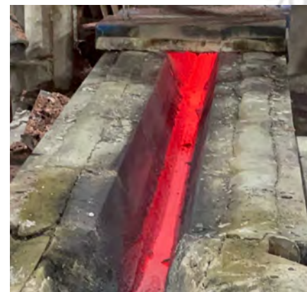
Precast inserts without sacrificial lining
