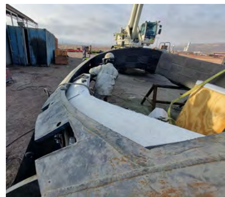
Installed METAL-ROK® Precast
