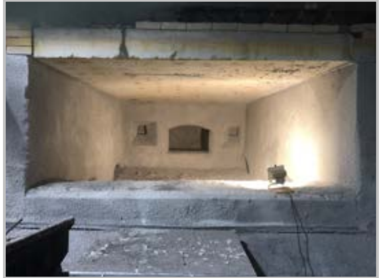
AFTER: QUICK-FIRE® 85 G installed
