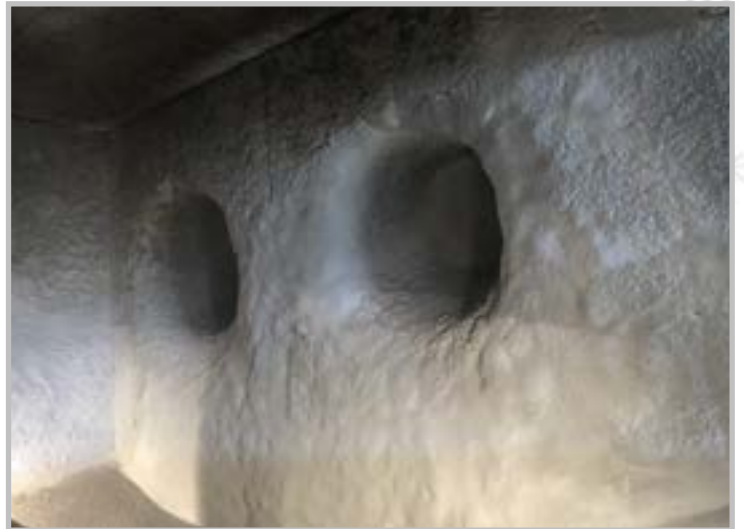
AFTER: QUICK-FIRE® 85 G installation completed
