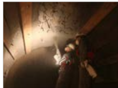
Shotcrete Installation
