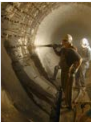
Shotcrete Installation
