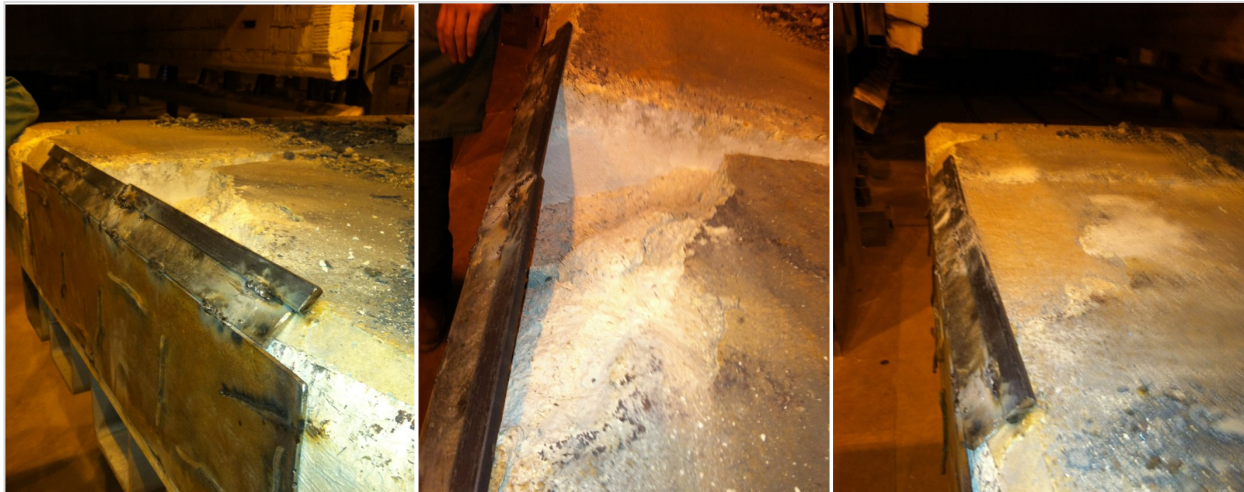
QUICK-FIRE® 65 perimeter repair
