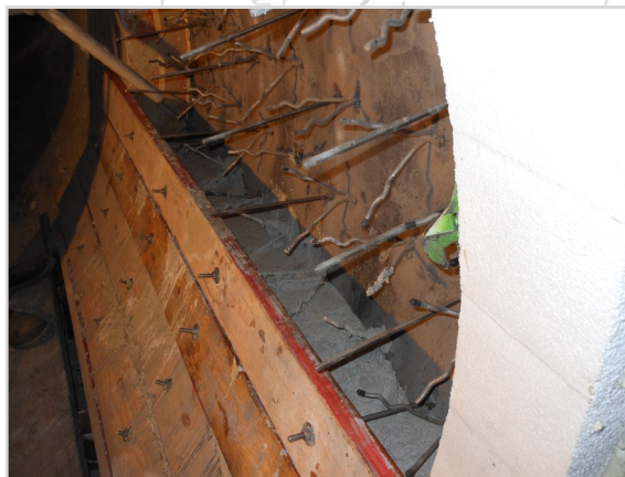
Rotary cooler with ARMORMAX® 70 SR
