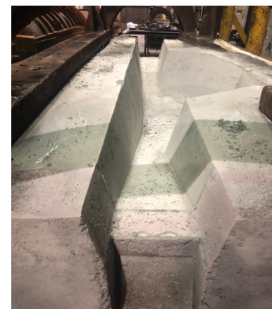
Blast Furnace Tilter
