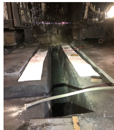
Blast Furnace Trough
