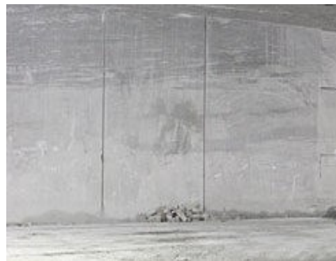
Sulfur Pit (After)
