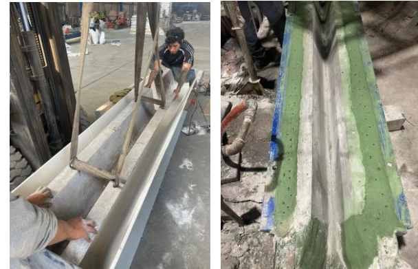
Installing precast launder segments
