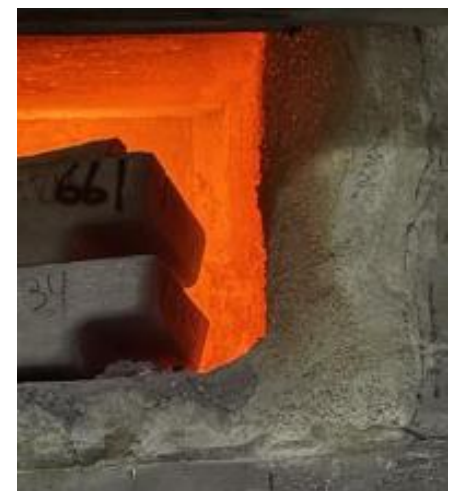
QUICK-FIRE® 84 G after 19 months of service
