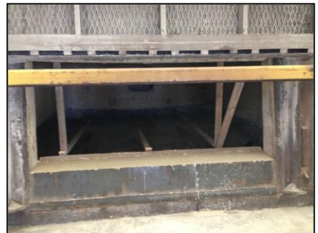
Installed sill
