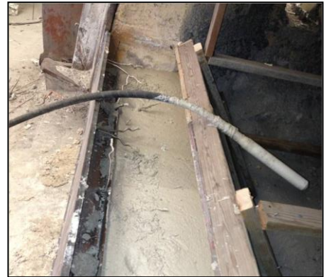
ARMORMAX® 70 AC installation
