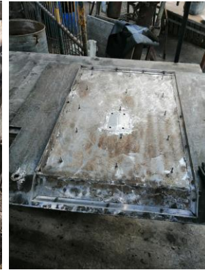
Shield cleaned, new screws as anchors and base for wire mesh
