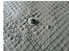
(Top left) initial layer against the splash shield. (Top right), mesh installed after initial layer. (Bottom left), casting second layer.
