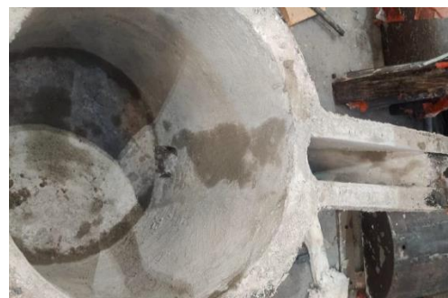
After fixing stone and coating with T-COAT® 7692M.
