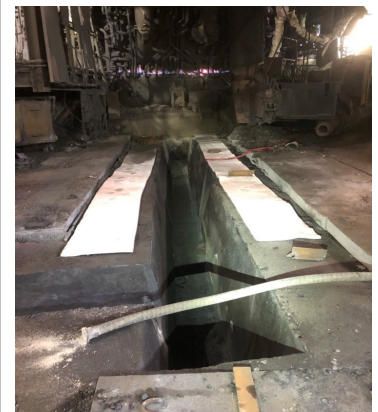
Blast Furnace Trough
