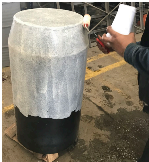
Application of the first coat of DRI-VIBE® DEFENDER 2 with roller. Mix of approximately 330 grams of powder for 99 grams of water
