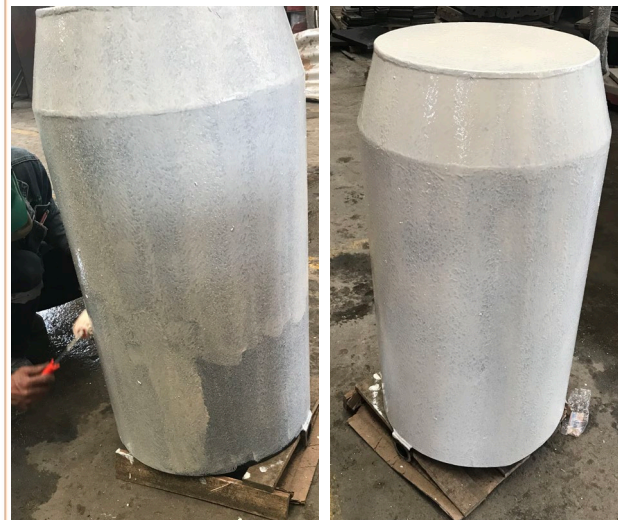
Left -Application of second quote / batch of DRI-VIBE® DEFENDER 2. Mix of approximately 330 grams of powder for 99 grams of water
