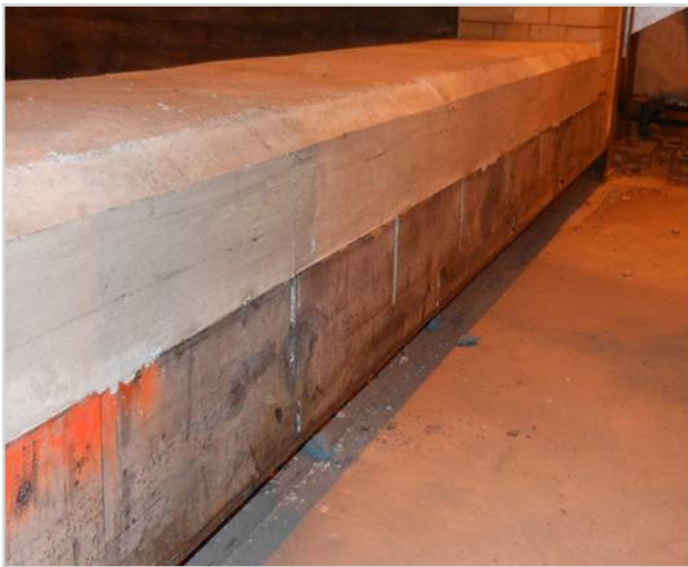
ARMORMAX® 70 SR in forge furnace sill
