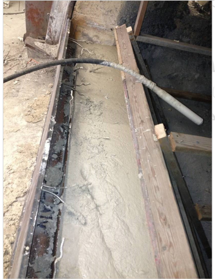
Aluminum reverb furnace sill cast with ARMORMAX® 70 AC
