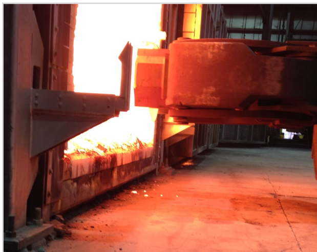
ARMORMAX® 70 SR forge furnace sill after 18 months in service
