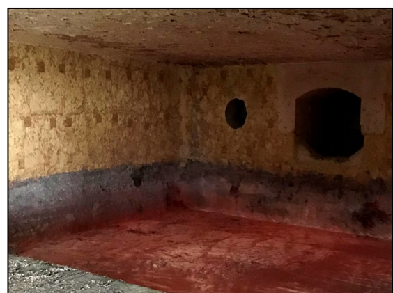
Reverb furnace after one year in service
