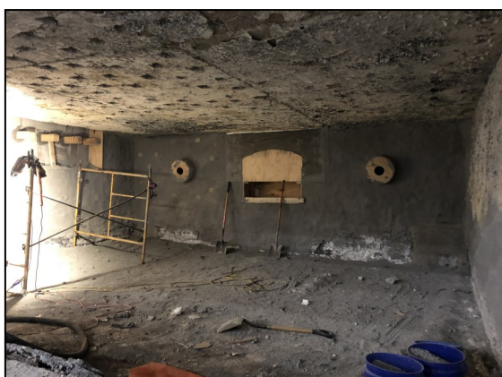
Reverb furnace fully gunned with REDIGUN
