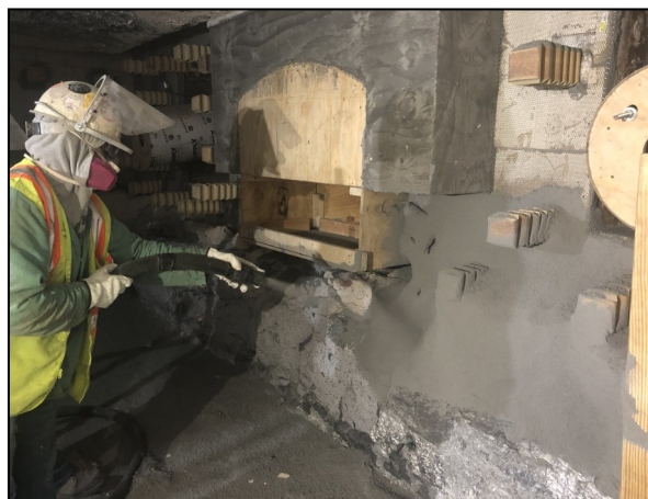
Installation on burner wall of 200,000 lb Reverb
