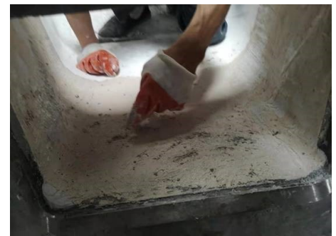
Spout repair using QUICK-FIRE® ONE 86
