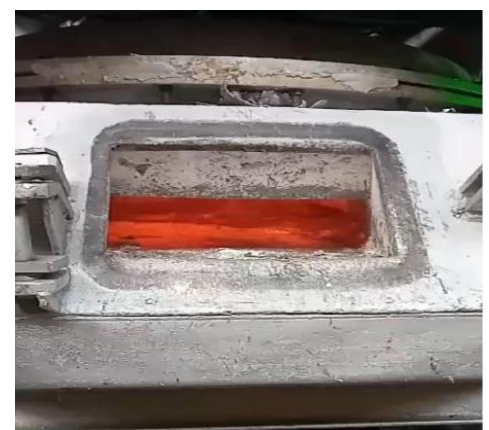
WAM® AL II after 6 months of operation
