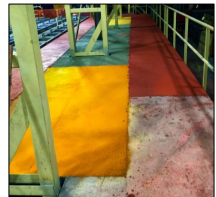
Completed TUFFLOOR® flooring sections
