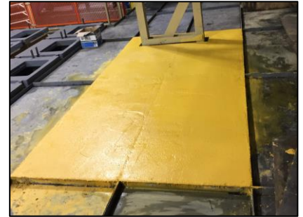
Installation of yellow TUFFLOOR® section
