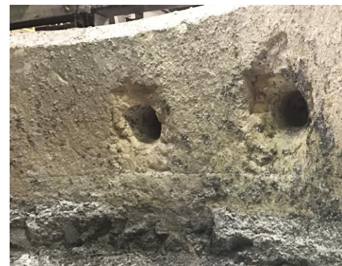
Furnace at current state
