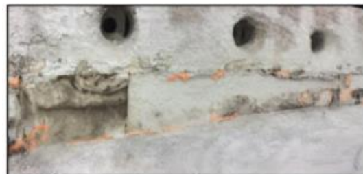
Top charge furnace before QUICK-FIRE® 85 G installation
