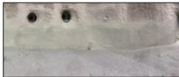
Top charge furnace after installation of QUICK-FIRE® 85 G
