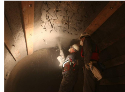
Shotcrete Installation
