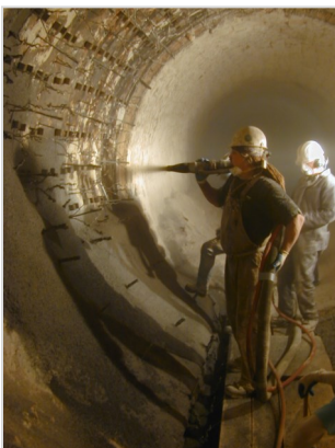
Shotcrete Installation
