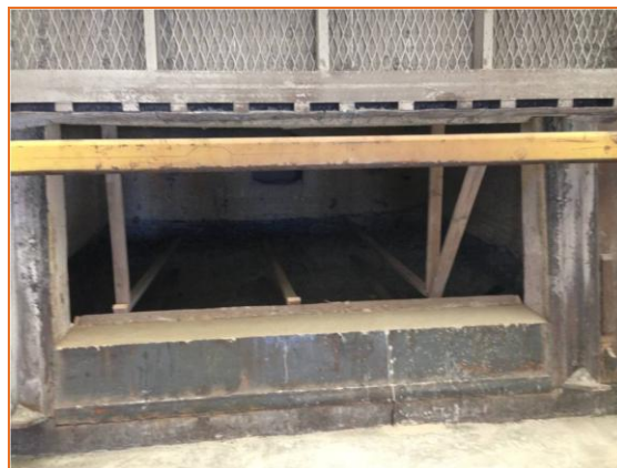
Installed sill
