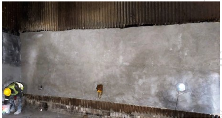
AFTER: QUICK-FIRE® PATCH M
