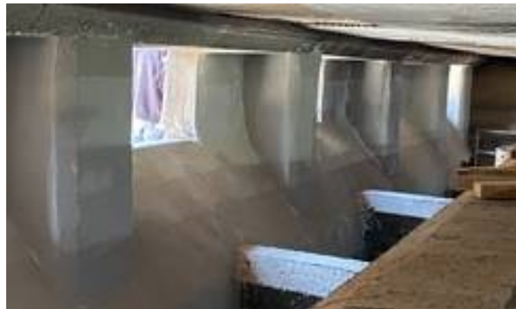
AFTER: QUICK-FIRE® PATCH M
