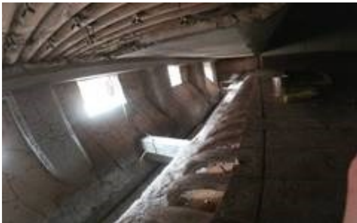
BEFORE: Installation of QUICK-FIRE® PATCH M
