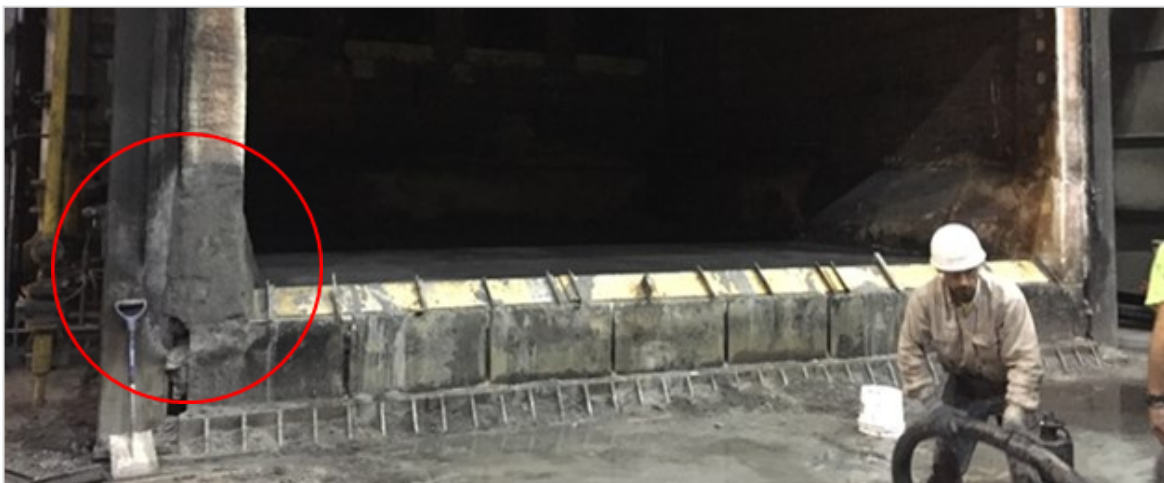
Lower jamb and curb wall repair with TUFFCRETE® 70X shotcrete
