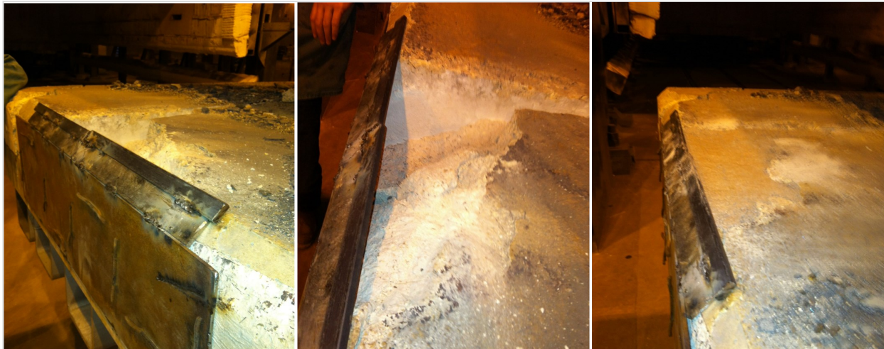
QUICK-FIRE® 65 perimeter repair
