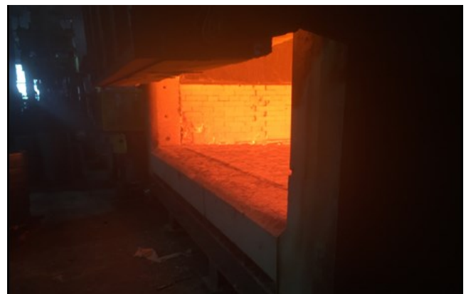
ARMORMAX® sill after 52 months in service
